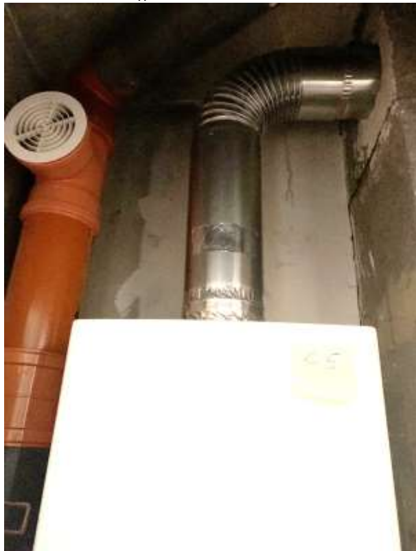
Raccordement B 11 & ventilation haute – lot 1 – C-5 - 0
