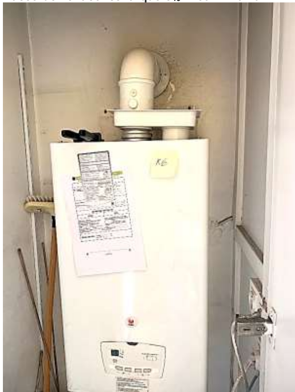
Raccordement concentrique C 13 – lot 1 - K6 - 0
