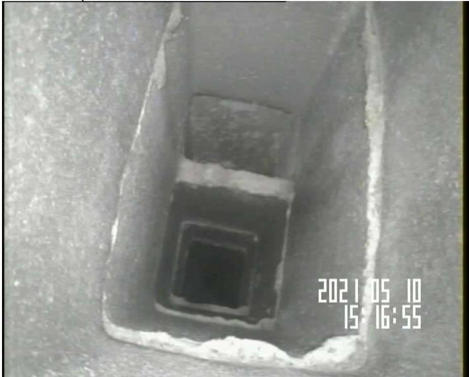
Shunt GB D2 passant de 200 x 350 – 200 x 125 mm → 200 x 200 – 125 x 200 mm
