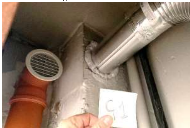
Raccordement B 11 & ventilation haute – lot 2 - G1 - 0
